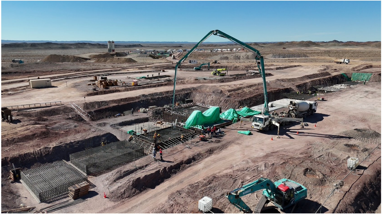
Figure 2: Bayan Khundii Project Process Plant Construction
