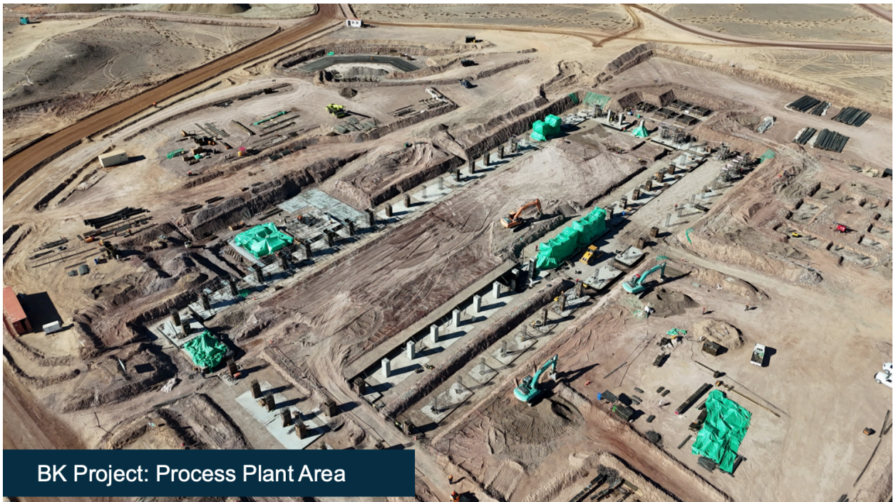
Figure 3: Bayan Khundii Project Process Plant Construction
