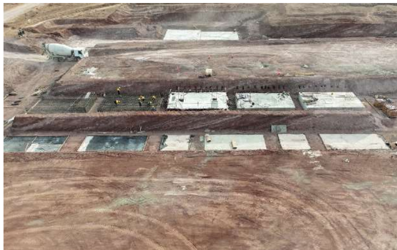
Process Plant Footings
