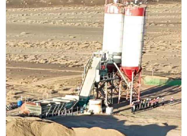
Concrete Batch Plant Establishment
