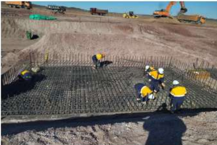
Foundation Rebar Installation
