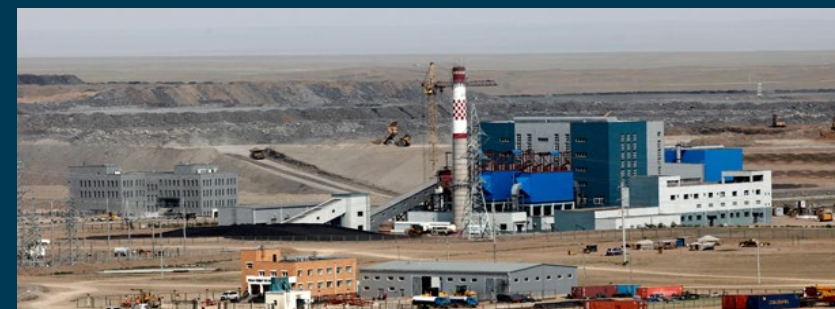
18MW UHG Power Plant – MCSI
