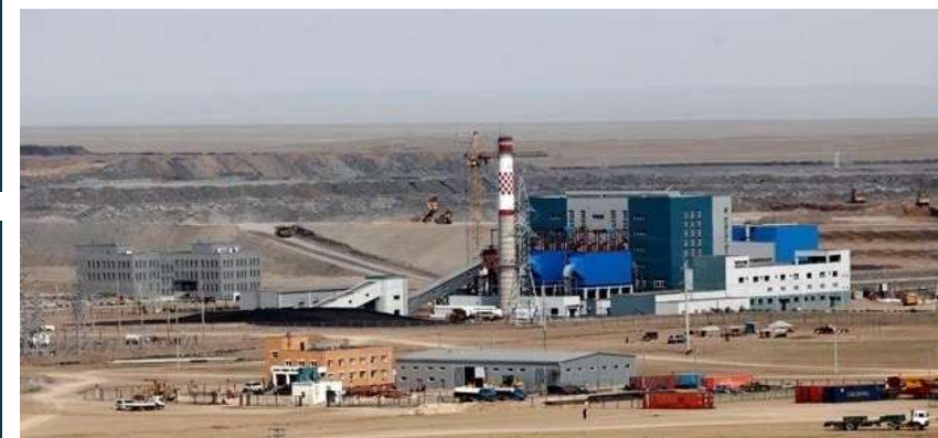
18MW UHG Power Plant – MCS I
