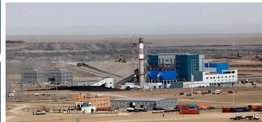
18MW UHG Power Plant – MCS I
