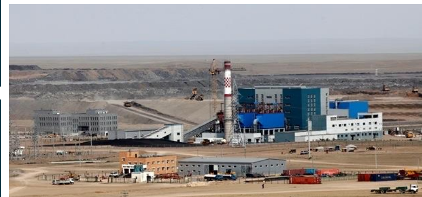
18MW UHG Power Plant – MCS I
