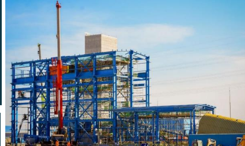
Oyu Tolgoi Underground Conveyor – MCS P
