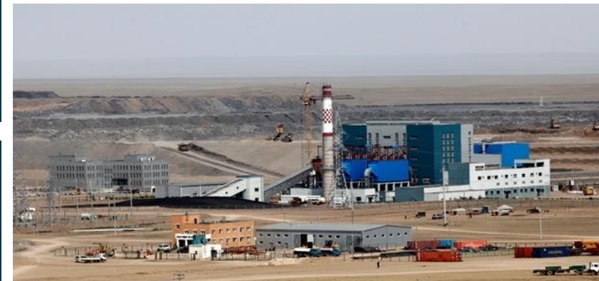
18MW UHG Power Plant – MCS I
