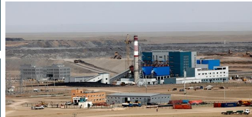
18MW UHG Power Plant – MCSI
