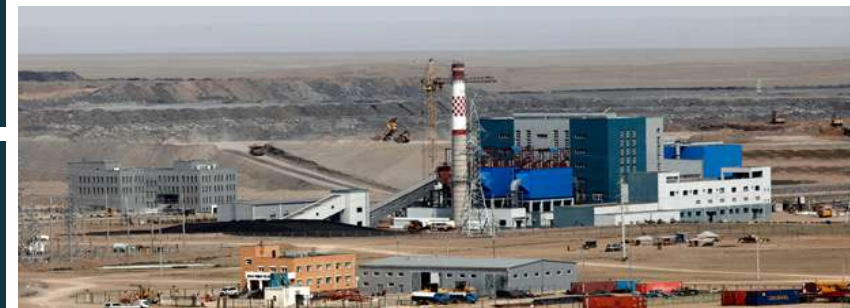
18MW UHG Power Plant – MCSI
