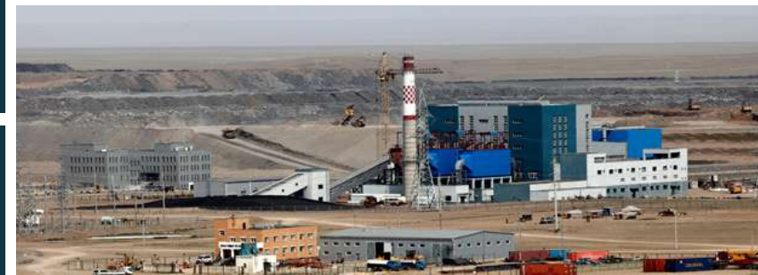
18MW UHG Power Plant – MCSI
