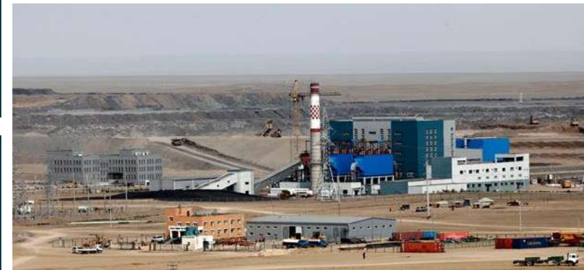
18MW UHG Power Plant – MCS I
